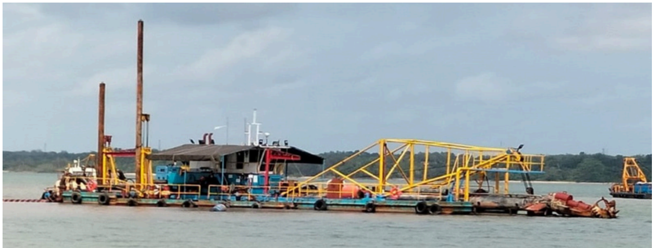
Cutter Suction Dredger
